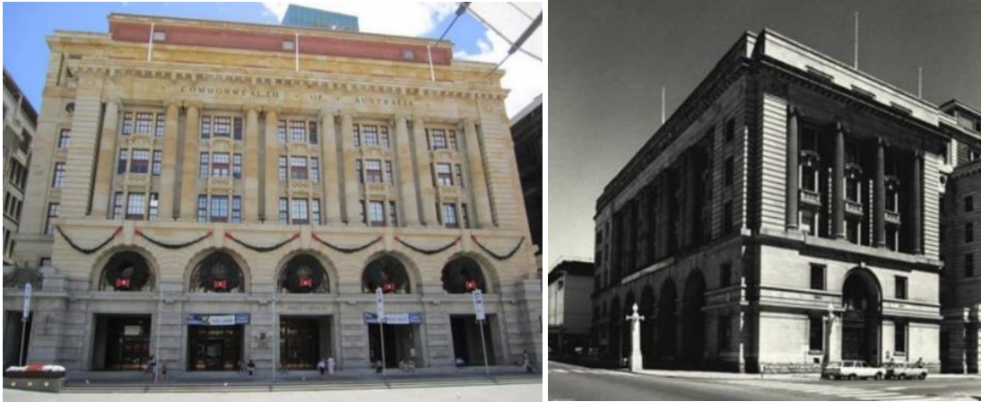
1912-1923 General Post Office (shown in 2011) and 1933 Commonwealth Bank (shown in 1986), both at Forrest Place, Perth (HCWA 01979, HCWA 02064).
